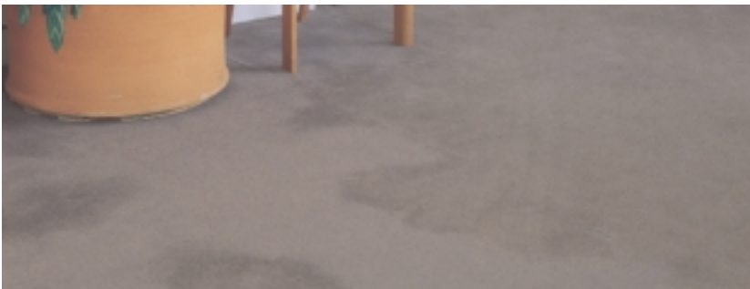
Photograph C - Watermarking, pooling and puddling
